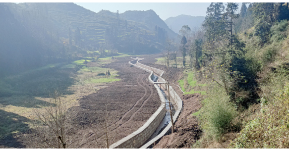
Water infrastructure project in Gouchangba Village, Putian Township
